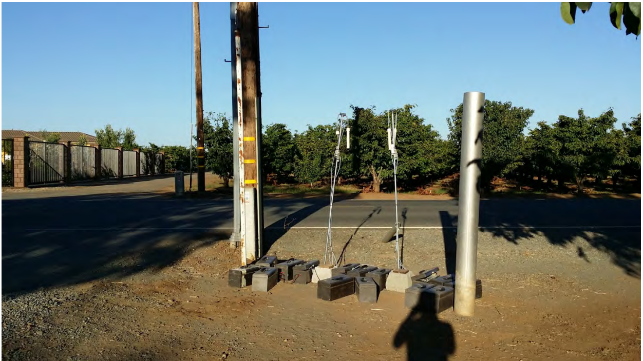
South East Corner – Facing East
