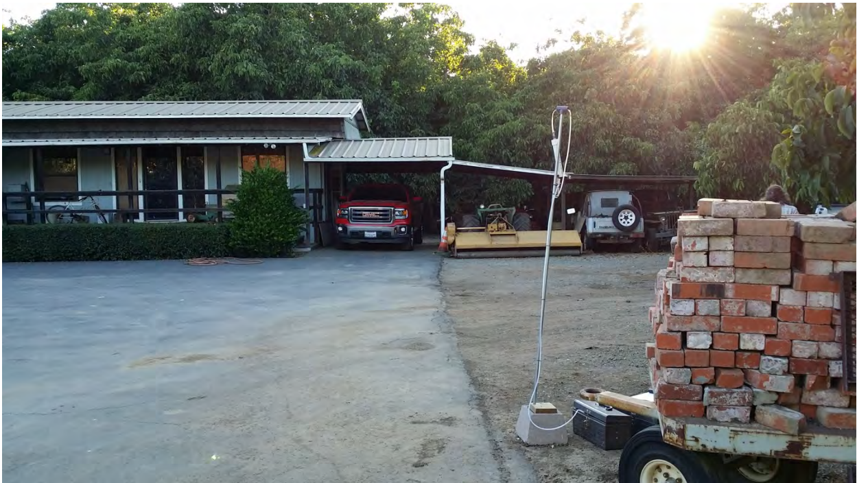
South West Corner – Facing West
