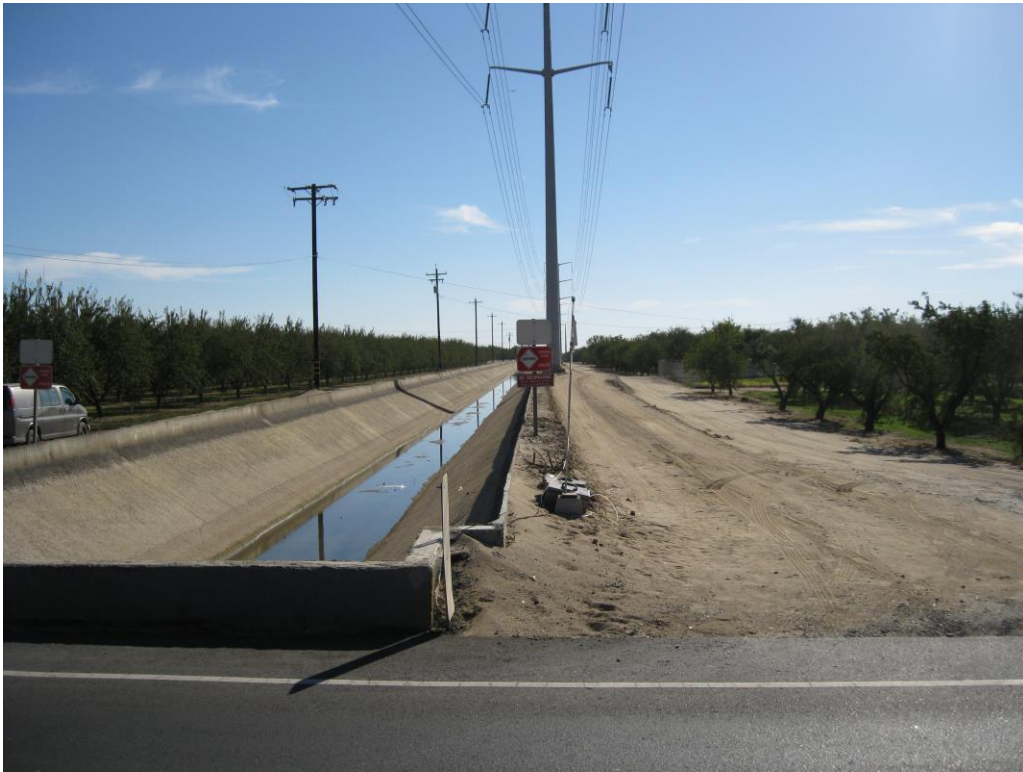
North West Corner Sampler Looking South
