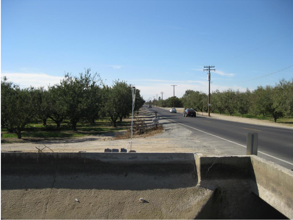
North West Corner Sampler Looking West
