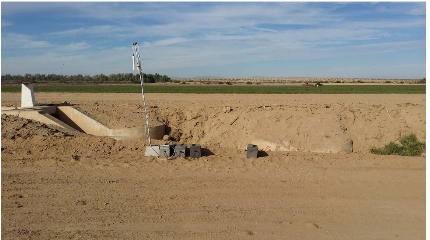
South West Site – Facing West
