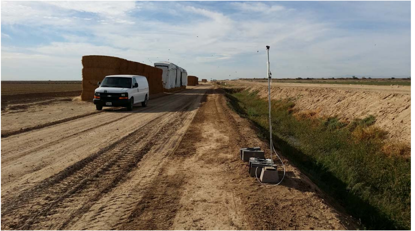
West Site – Facing South
