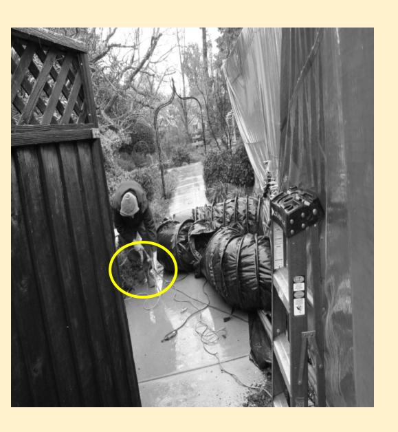
**Aeration duct had** disconnected from the eave and fan was still running. The inspector observed the licensee unplugging the aeration fan
