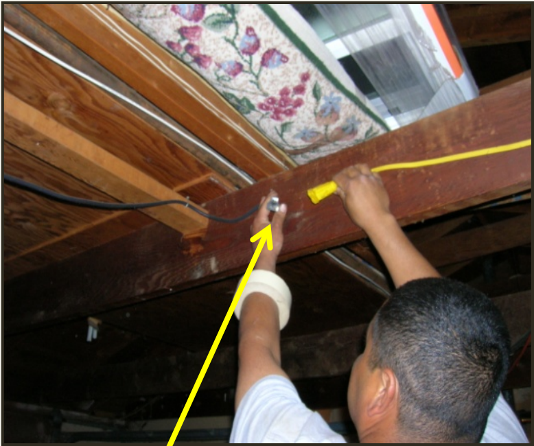
Licensee is disconnecting the electrical power cord to disable the automatic garage door opener.
