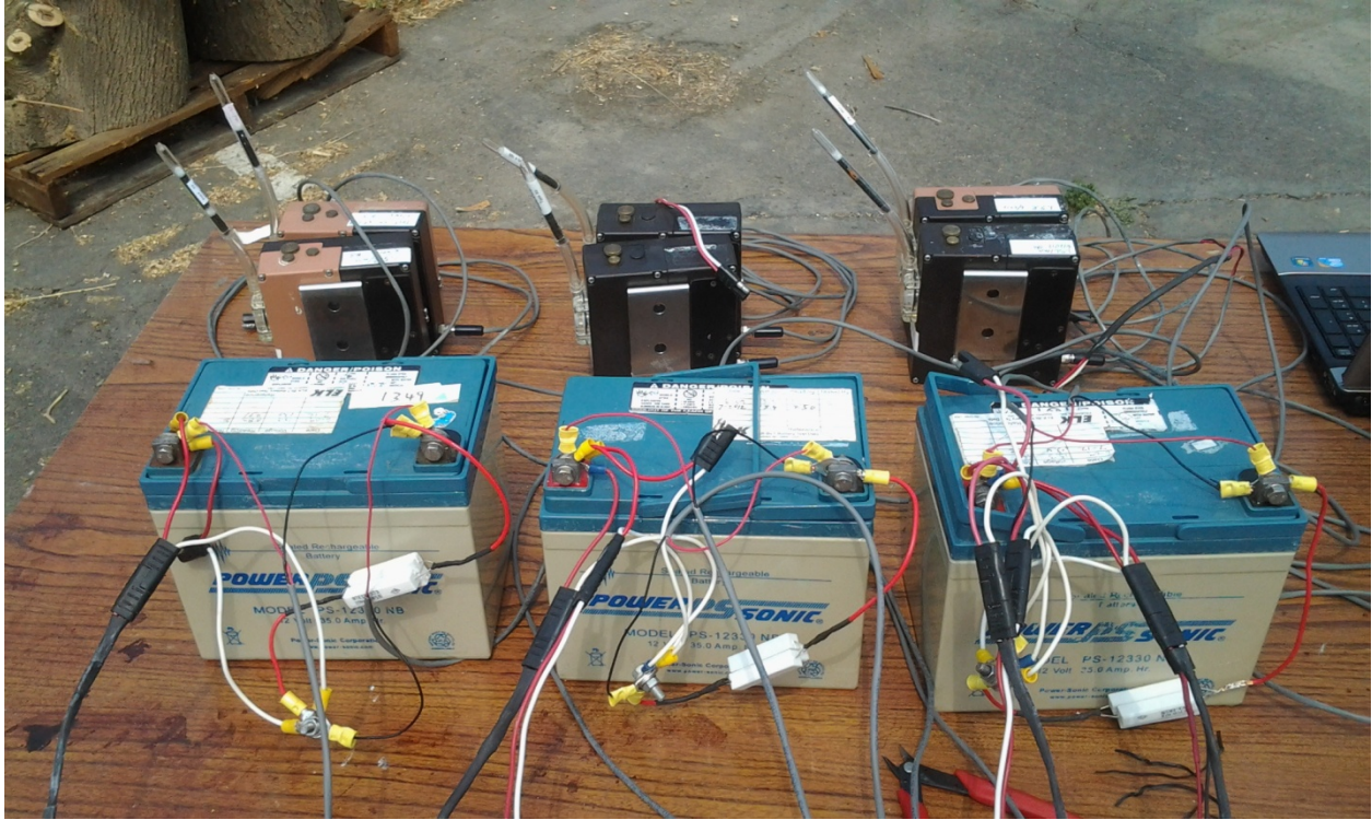
Picture 5. Batteries connected to the two SKC Aircheck pumps.
