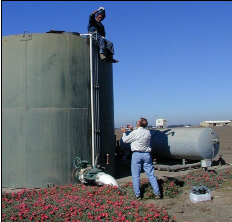
Figure 15. Example of unpressurized storage tanks. Samples were collected from the inflow into the tank from the small pipe going up the side and entering at the top by reaching inside the tank through the access port.
