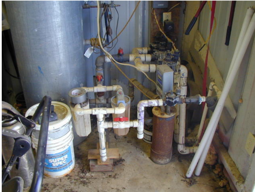
Figure 5. Locating the sampling port is not always easy. In this case, a faucet outside the shed wall to the right (not shown) could be used as the sample port as long as the proper valves were opened, negating the need to collect samples through the Schrader valve.
