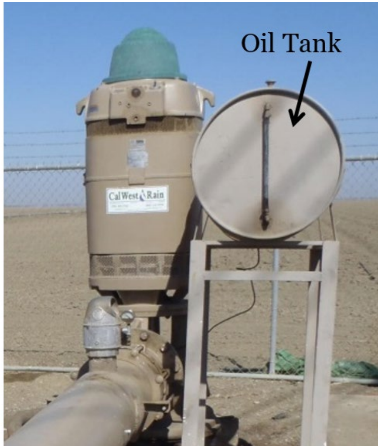
Figure 11. Oil tank for a turbine pump, not to be confused with a chemigation system.
