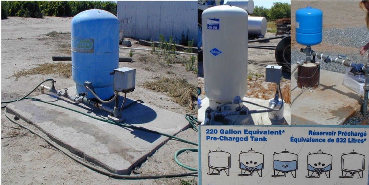
Figure 14. Examples of fixed bladder tanks. Note that there is only one pipe connected to the tank itself. Samples can be collected from the faucet on the left after the hose has been removed.
