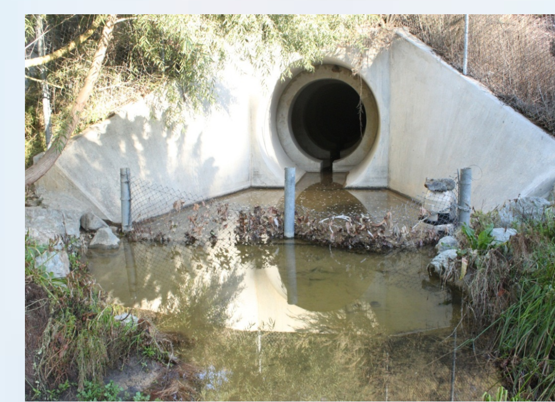
Figure 1. Storm drain entering pond
